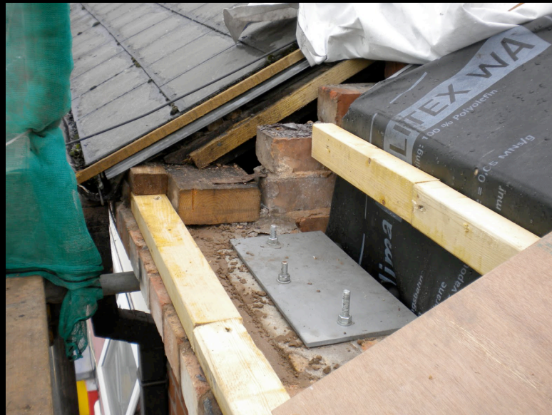
Roof pod footing to terrace walls.
