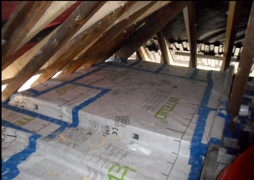
Preparation of joints at roof, first floor and ground levels for new bay window.
